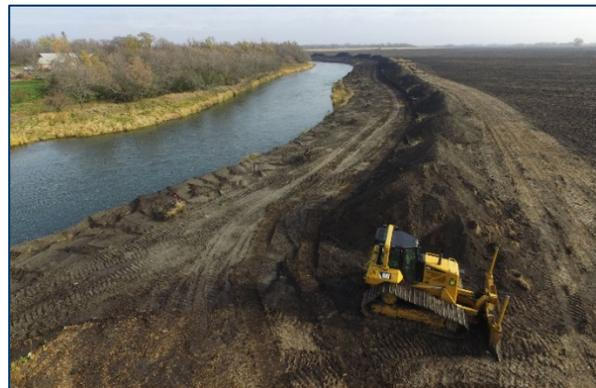
*From left: Day 1 of a streambank restoration project on the Otter Tail River in Wilkin County shows, at right, the field that was eroding into the river. A \$135,000 Clean Water Fund grant restored a 1,200-foot stretch of the bank. Heavy equipment was at work on Day 9. . Photo Credits: Wilkin SWCD*
