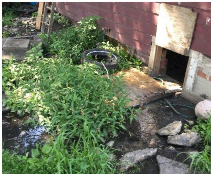
*Septic tank overflowing with sewage due to damage or tile blockage in Myrtle.*
