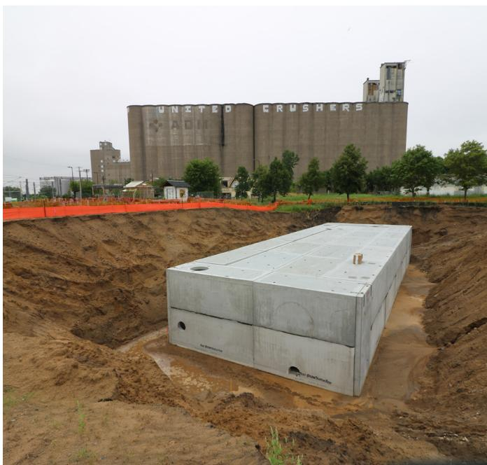
*The storage tank beneath the main basin can hold up to 206,575 gallons of treated runoff.*
