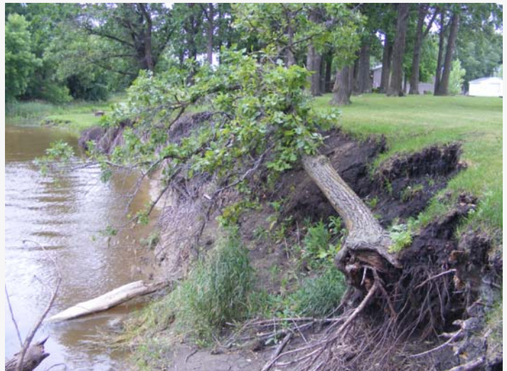
Trees being undercut along Thief River
