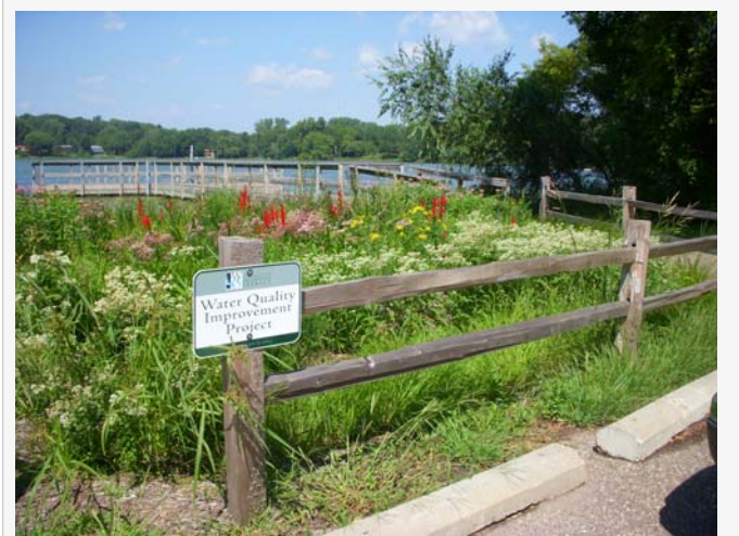
This recently completed shoreline restoration is an example of the types of features that will be installed as part of this project.
