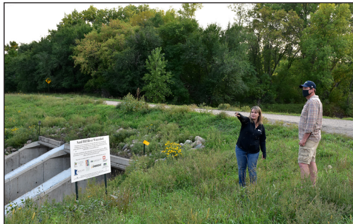
Sand Hill River Watershed District Administrator April Swenby showed BWSR Board Conservationist Darren Mayers elements of the rock riffles and rock arches project in September 2021 on a stretch of the river east of Beltrami. Photo Credit: Ann Wessel, BWSR
