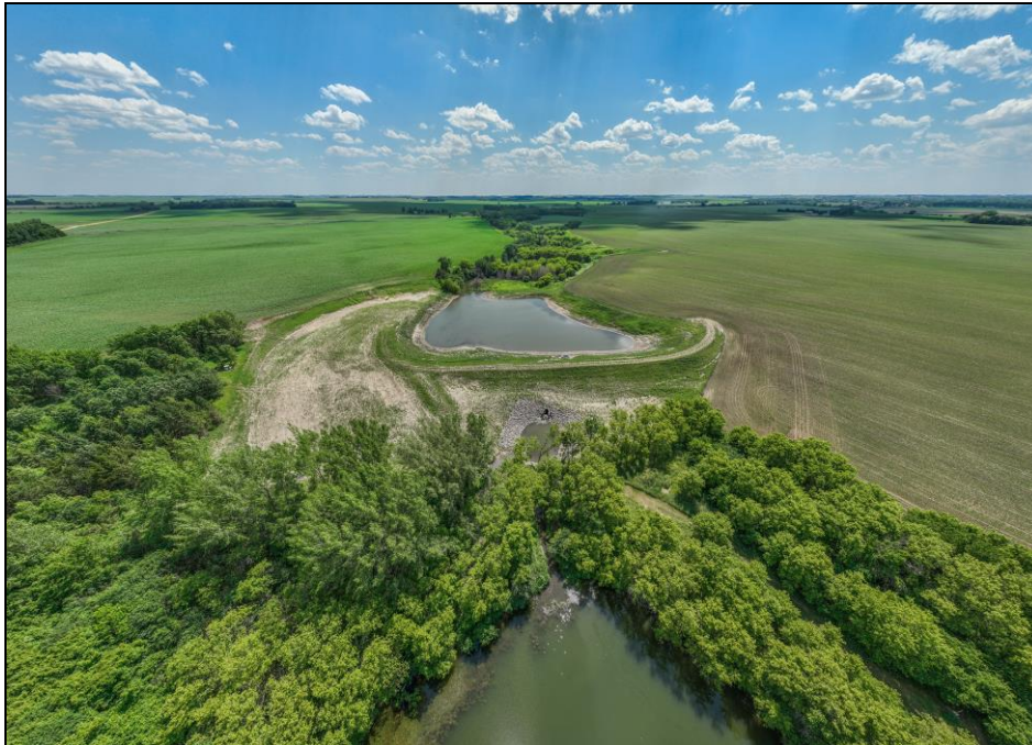
Springdale 19 Grade Stabilization (Lyon County)
