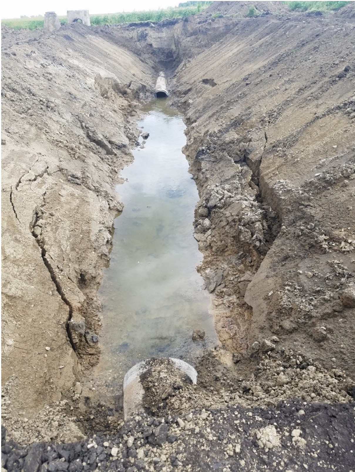
Figure 2: Temporary Modification at Sinkhole (Approximately Station 35+00)
