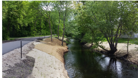
From left: By late summer 2016, native plants grew along Shingle Creek WMC's Connections I stream restoration. Erosion control fabric covered native vegetation planted in spring 2016. A dense tree canopy appears along a segment of the planned Connections II project. Photo Credits: Shingle Creek WMC
