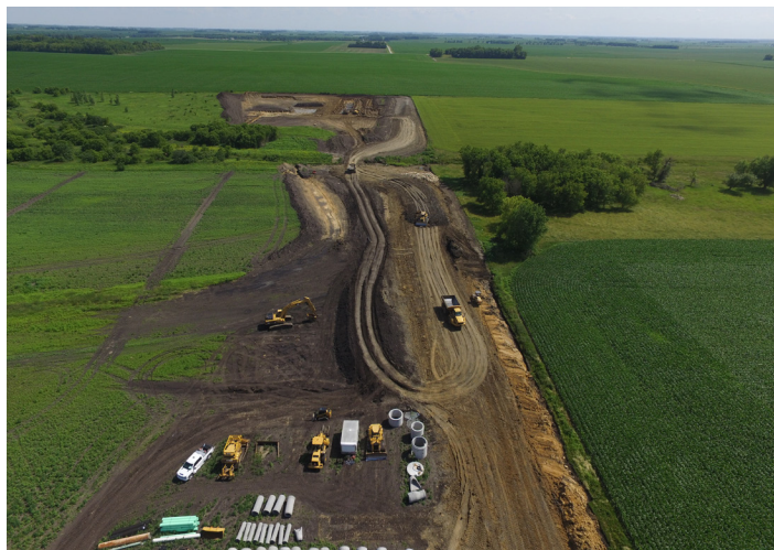
BWSR Board tour attendees visited a water storage structure in Mower County's Dexter Township (shown under construction above). The completed project (below) is estimated to reduce phosphorus by 194 pounds per year and total suspended solids by 126 tons.
