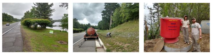
Left: Inlets to underground sediment collectors lie just off Crow Wing County Road 66 at Big Trout Lake. Middle: Maintenance involves periodic sediment removal. Right: Crow Wing SWCD Manager Melissa Barrick and AmeriCorps intern Reece Boucher lend scale to a sediment collector.
