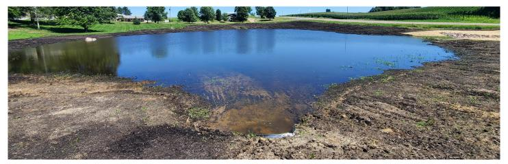
Contractors in summer 2020 excavated more of the wetland to increase flood storage, and installed a culvert connecting it to the upper watershed.
