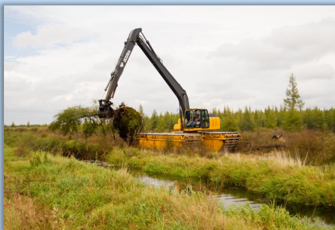
Filling of old drainage ditch to restore hydrology.
