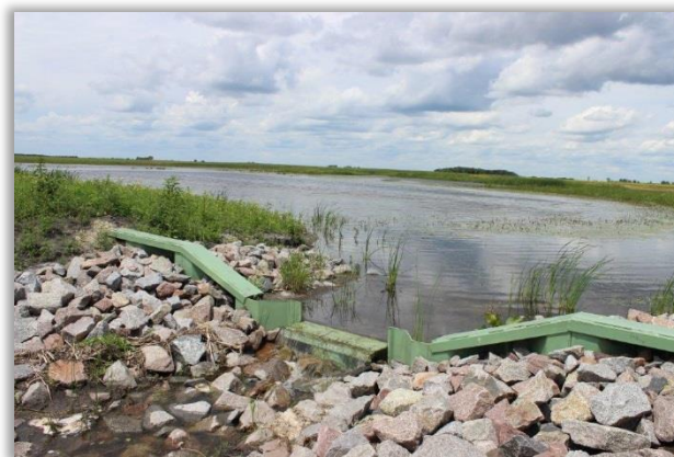
The Ellefson Wetland Restoration in Norman County.
