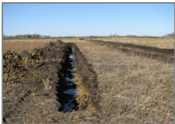
Figure 12. Tile Investigation Trench
