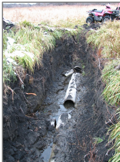
Figure 1. Removing “Blocking” Subsurface Drainage Tile
