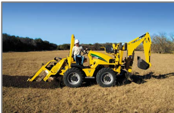
Figure 6. Supplemental Trenching to Aid in Destroying Subsurface Tile Within Sloped Wetland Settings
