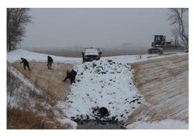
Erosion & sediment control applied during snowstorm as project nears completion.
