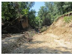
One of the major projects was an earthen dam that blew out during the heavy rainfalls, sending approximately 5,500 tons of sediment downstream and leaving unstable vertical banks behind. Constructed in the 1970s, to provide rate control for an upland watershed to the Cannon River, there was not enough funding available to replace the dam. Those banks were a safety risk in the park, though, which made repairs on the public land eligible for FEMA funding.
