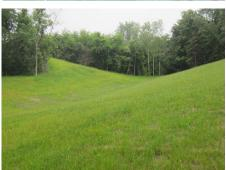
The SWCD graded the vertical banks into gentle slopes and installed permanent geotextile turf reinforcement mats to hold soil in place, and then reestablished site vegetation using topsoil, native seed and more erosion control blankets.
