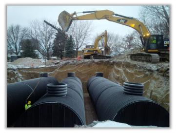
Phase two of the project installed three storage tanks that will be used to hold water.
