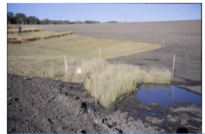
Prevegetated mats, erosion fabric and straw bales stabilizing a swale
