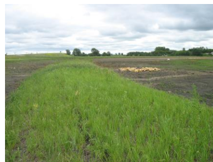
Wetland embankment vegetated with a native construction mix
