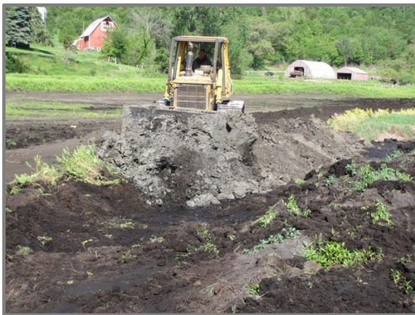
Figure 2. Shallow Ditch Being Filled
