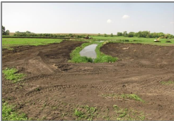
Figure 1. Construction of an Earthen Plug Across Drainage Ditch
