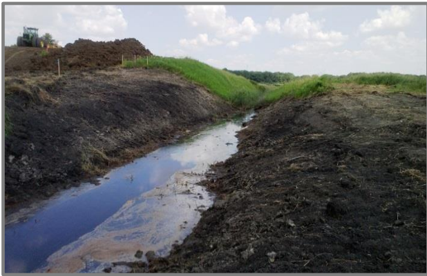
Figure 9. Ditch Area being Stripped Prior to Plug Construction
