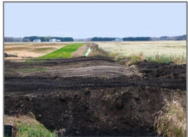
Figure 12. Finished Ditch Plug with Crown in Middle
