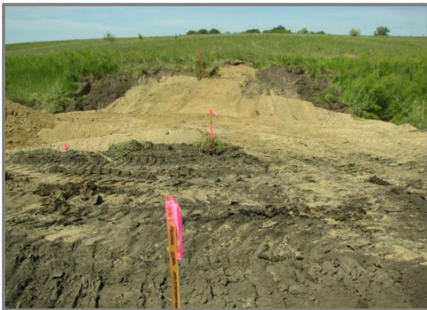
Figure 10. Ditch Plug under Construction
