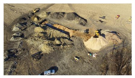
A drone image depicts a woodchip bioreactor under construction in Faribault County. Photo Credit: Fairbault County
