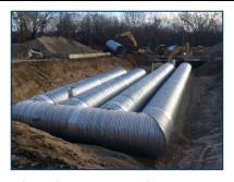
FROM LEFT: Most of the work to construct a cistern and a series of pipes under the softball field and part of the parking lot at Upper Villa Park in Roseville was completed in late fall 2015. The softball field at Upper Villa Park in Roseville is now irrigated with rainwater collected in an underground cistern. A series of underground pipes perforated with thousands of holes will allow rainwater to seep into the ground. Photo Credits: Capitol Region Watershed District
